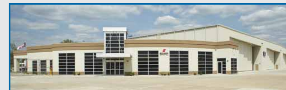
As of April, most of the exterior was done, thus leaving the contractors to work on finishing the shell of the new Elliott Aviation Facility. Here's the final look for the exterior.
