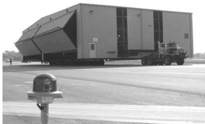
Moving the 7,579 sq. ft. hangar.
